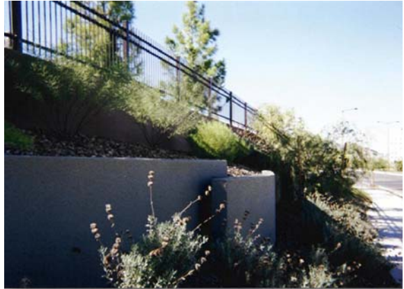
Figure 50-26.4-B: Retaining wall terracing and articulation
