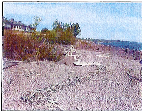
Figure 7 – west side of Ledges Townhomes looking east
