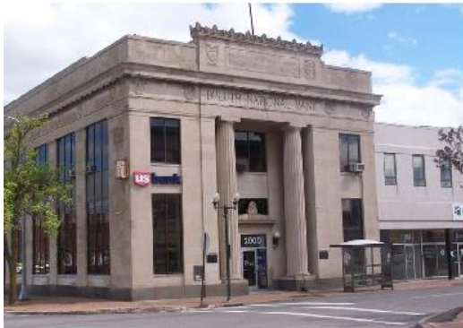
Example of Corridor Building II
