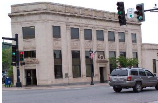
Example of Corridor Building II
